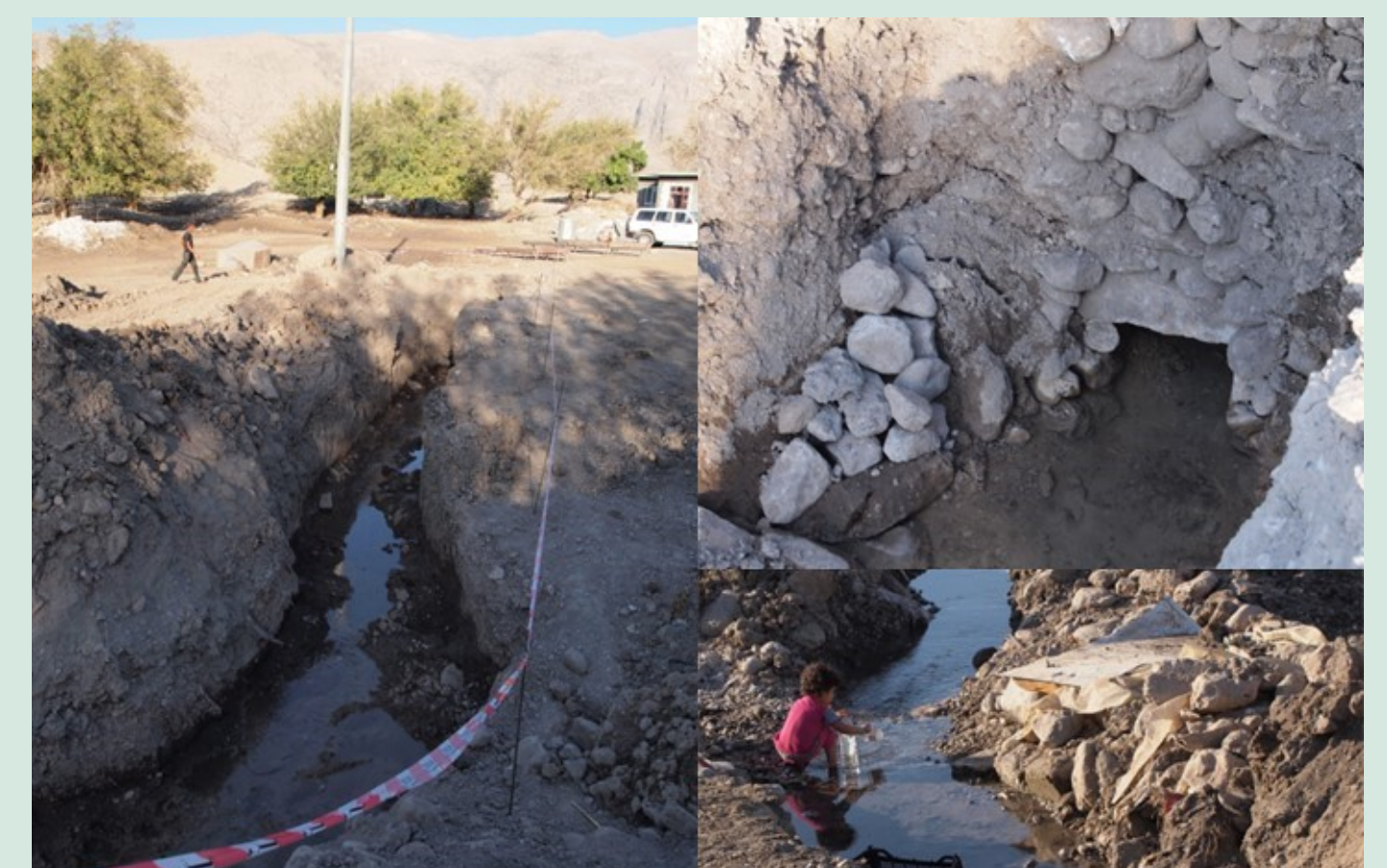
A qanat being renovated in Sulaymaniah Governorate, Kurdistan Region of Iraq. Photo: Lina Eklund 2012
