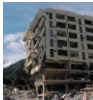
Damage by debris flows in two buildings on the alluvial fan of San Julian River (right picture is a closer view of the building in the background in left picture)
