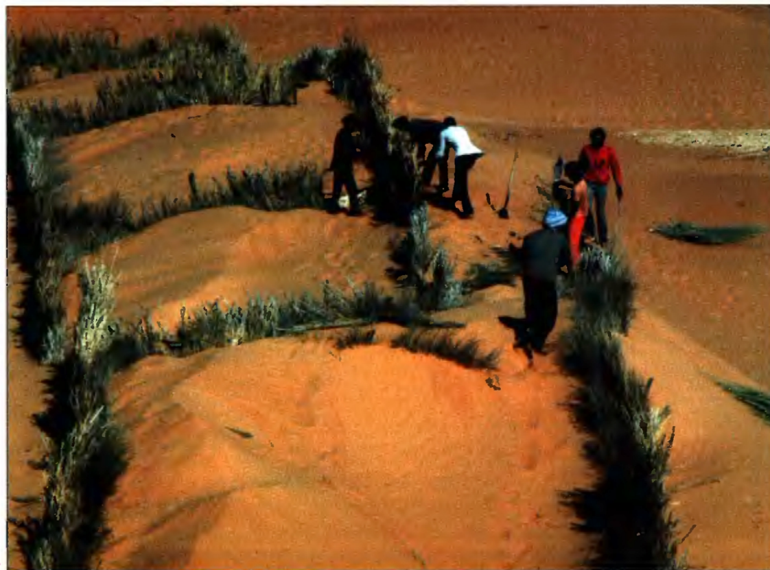
Mauritania — Dune fixation with windbreak fences made from branches of Balanites (FAO/R. Faidutti)
