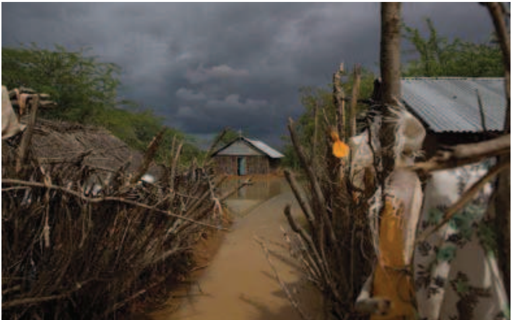
Recent floods in Kenya drove villagers from their houses, destroyed crops and livestock and caused severe soil erosion; B.Bannon/UNHCR
