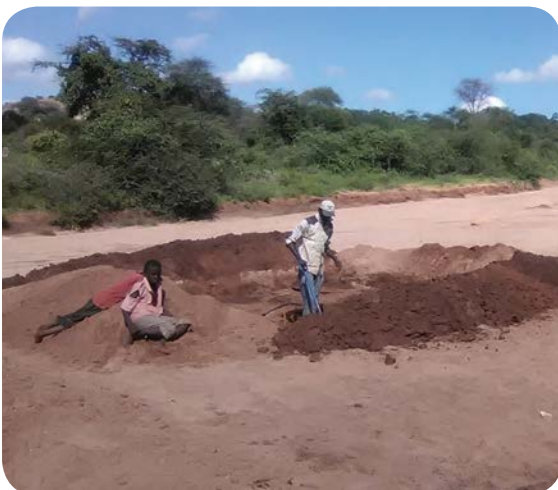
Constructing sunken sand dams (Photo: Joseph Ngodi)
