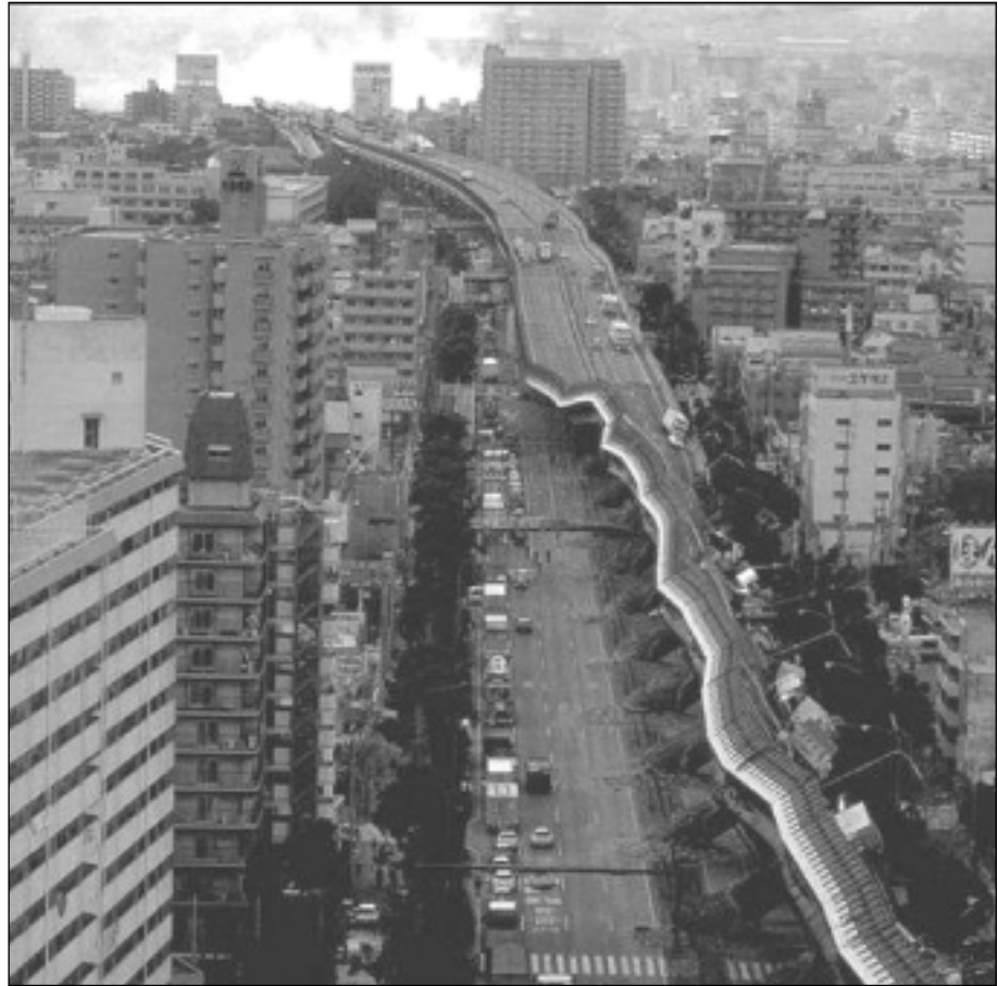
Figure 2. Spectacular collapse of the Hanshin Expressway as a result of the 1995 Kobe earthquake (Reproduced from the Kobe Geotechnical Collection, University of California, Berkeley).
