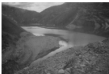
Figure 17. Outflow from the excavated channel over the dam crest.
